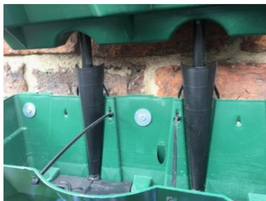
A length of 13mm irrigation pipe which is easily cut with pipe cutters is fitted onto the overflow spouts on the underneath of the Vertical Planter. The length is dependant on the planter spacing's, 15-20cm lengths are normal but the pipe should be long enough to go into the funnel by 5 cm. This will flow the water directly into the funnels and guarantee alignment so the water is not spilled out.
